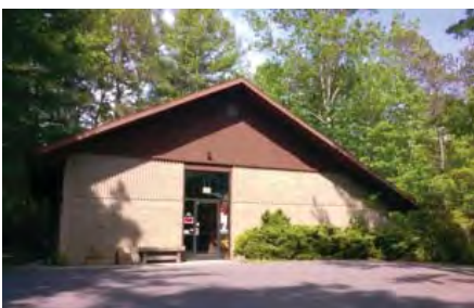
Williamson Creek Community Center
