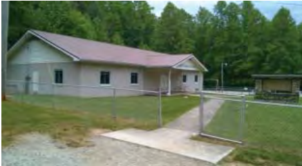
Quebec Community Center
